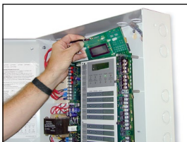
The DACT/Dialer installs behind the front panel display.
